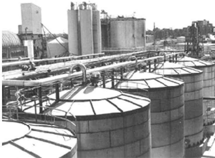
Figure 4. The continuous fermentation train previously operated by Williams Energy in Peoria, IL.
